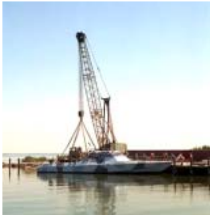
Land crane on pier
