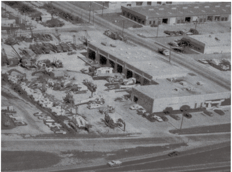
Kirkpatrick & O'Donnell Construction Equipment, Dallas, Texas
