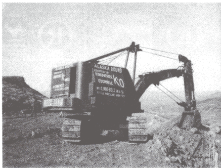
First Kirkpatrick Excavator delivered to the Alaska Pipeline
