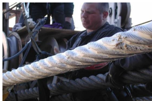
Hoover Dam – 76mm -Being coated with Dynagard E™
